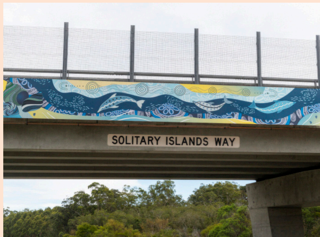
↓ Artwork installation Arararra interchange southbound. Photo via NSW Transport
